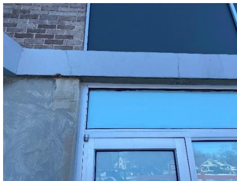
Figure 2 Concrete base cracking example at 1965 Building
